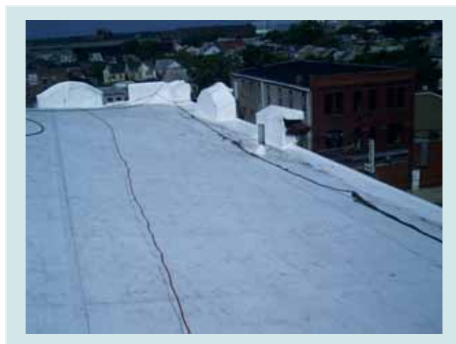
544 Chestnut Ave. - New Roof
