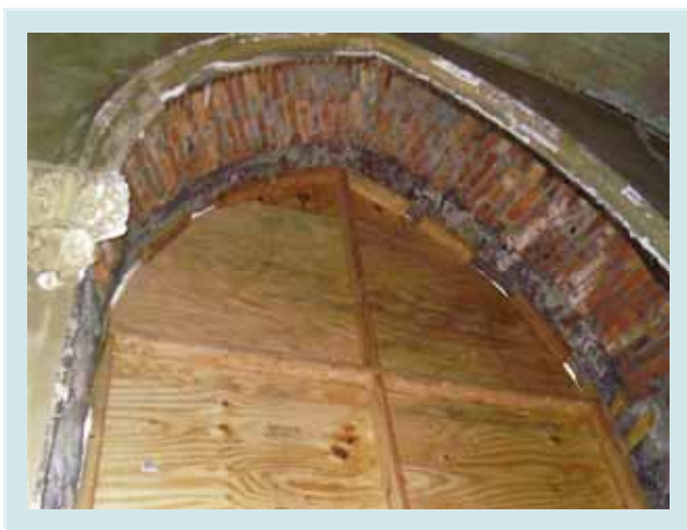
ICC Campus—4 Tower Windows
