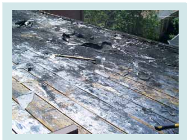
544 Chestnut Ave. - Removal of 12 layers of roofing materials
