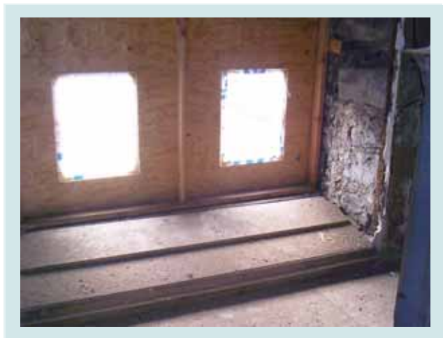
ICC Campus—4 Tower Windows
